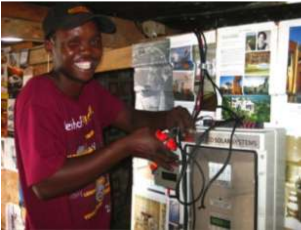
Figure 3. Hub Operator Installing a solar system
